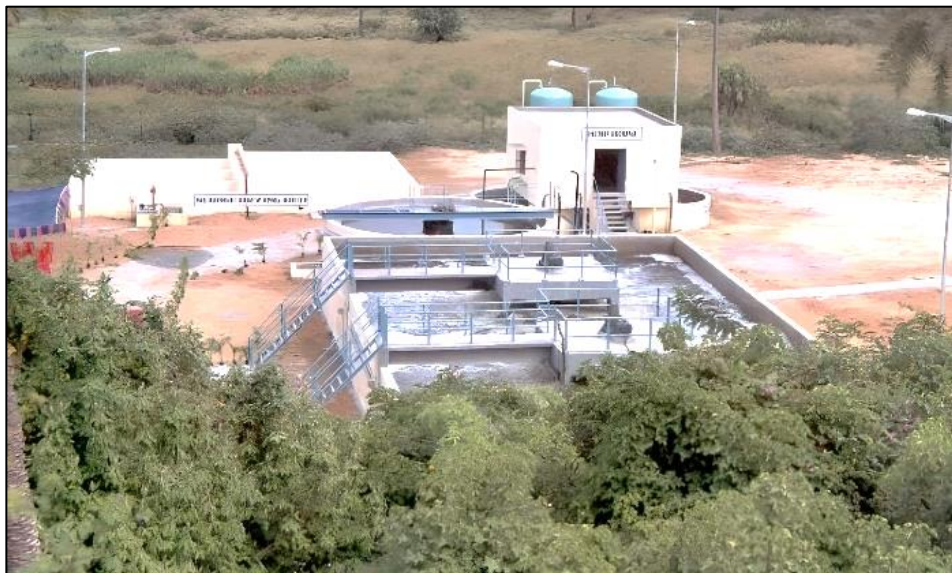
Overview of Sewage Treatment Plant
