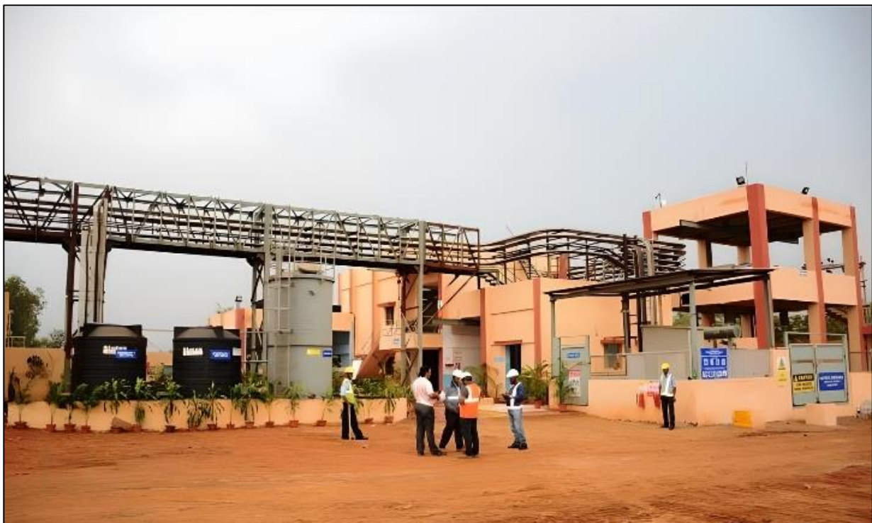
Acid dyke area with safety Arrangements
