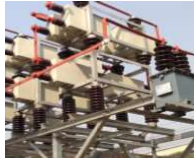
HT Capacitor banks of voltage levels from 3.3 kV to 132 kV
