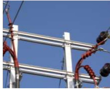
Cable termination kits, insulating sleeves, shrouds etc.
