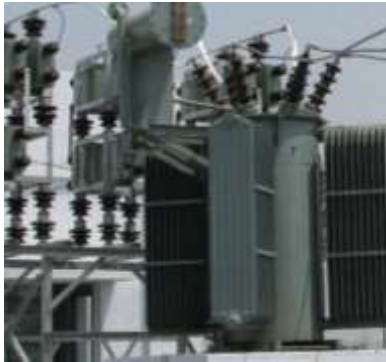
HT Passive Harmonic Filters
