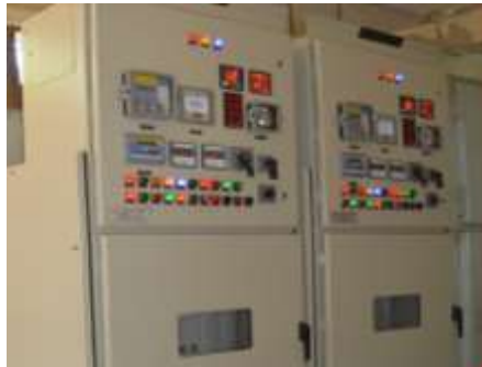
Indoor MV Switchgears upto 33 kV
